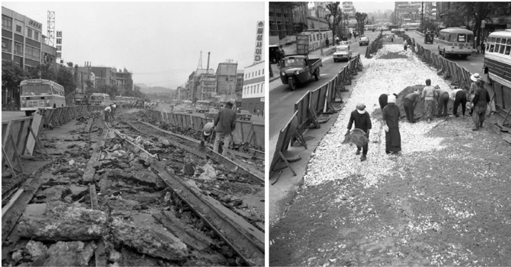
[Figure 12] Demolition of Tram Tracks
