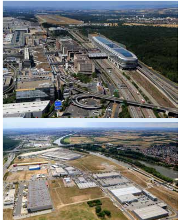
Figure 3. FRA Central airport city and Mönchhof logistics park Source: Fraport
