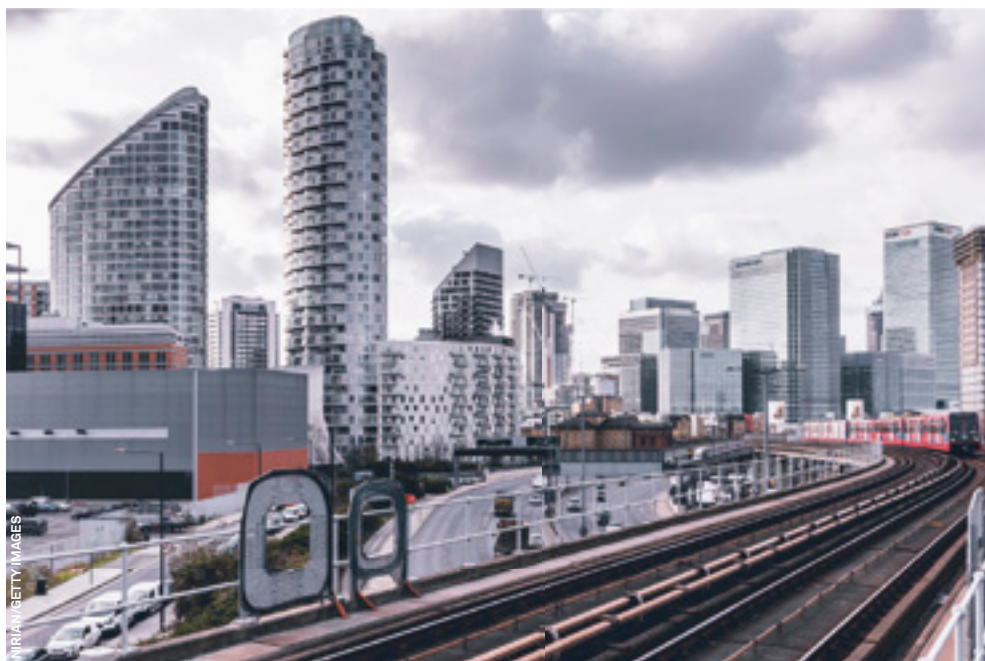
London’s verticalisation occurs in central areas and those that are well connected by public transportation (photo: Poplar Docks and Canary Wharf).
