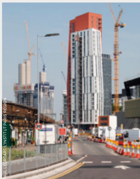
Tall buildings in construction at Nine Elms.
