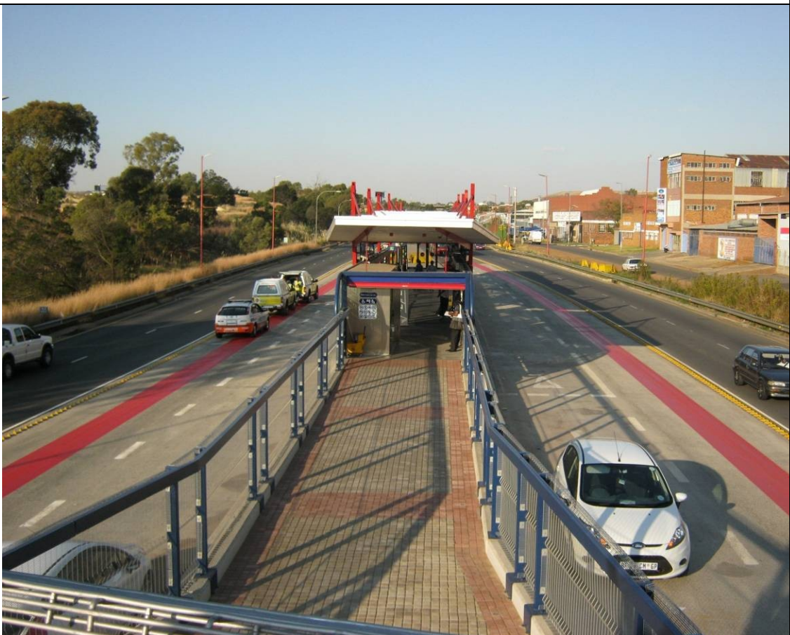
Rea Vaya Meadowlands Depot: administration building
