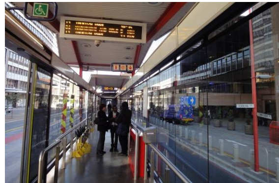
Pict. 2: Well-designed and technically well equipped bus stations
