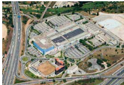
Centre comercial / Centro comercial / Shopping centre. Baricentro
