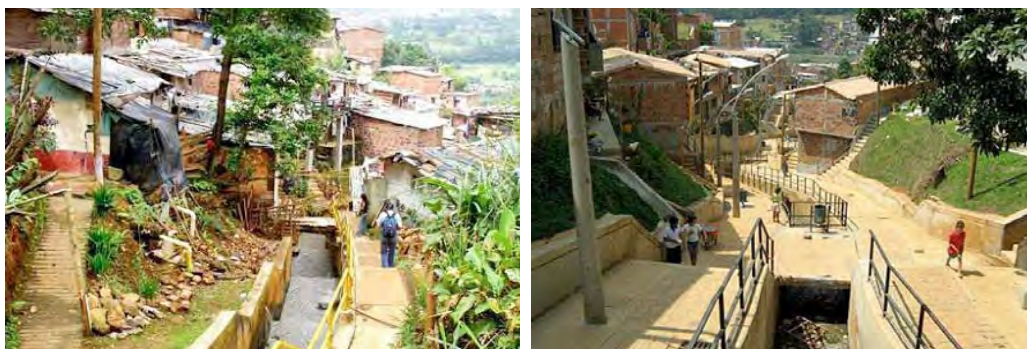
Medellin - before and after upgrading
