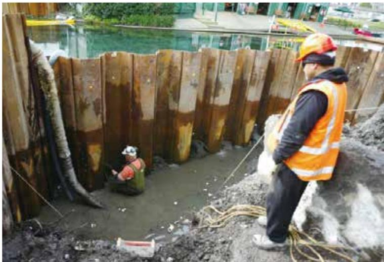
在为安堤瓜街大桥建造新的桥台时，工人们加固了挡土墙，把水挡在海湾外。SCIRT 负责重建城市的“基础性设施”，包括供水系统，地下设施和路面交通。Engineers reinforce retaining walls to keep water at bay while building new abutments for the Antigua Street bridge. SCIRT is responsible for rebuilding the city's "horizontal" infrastructure, including water systems, underground utilities and roads. (David Killick/*Citiscopes*)
